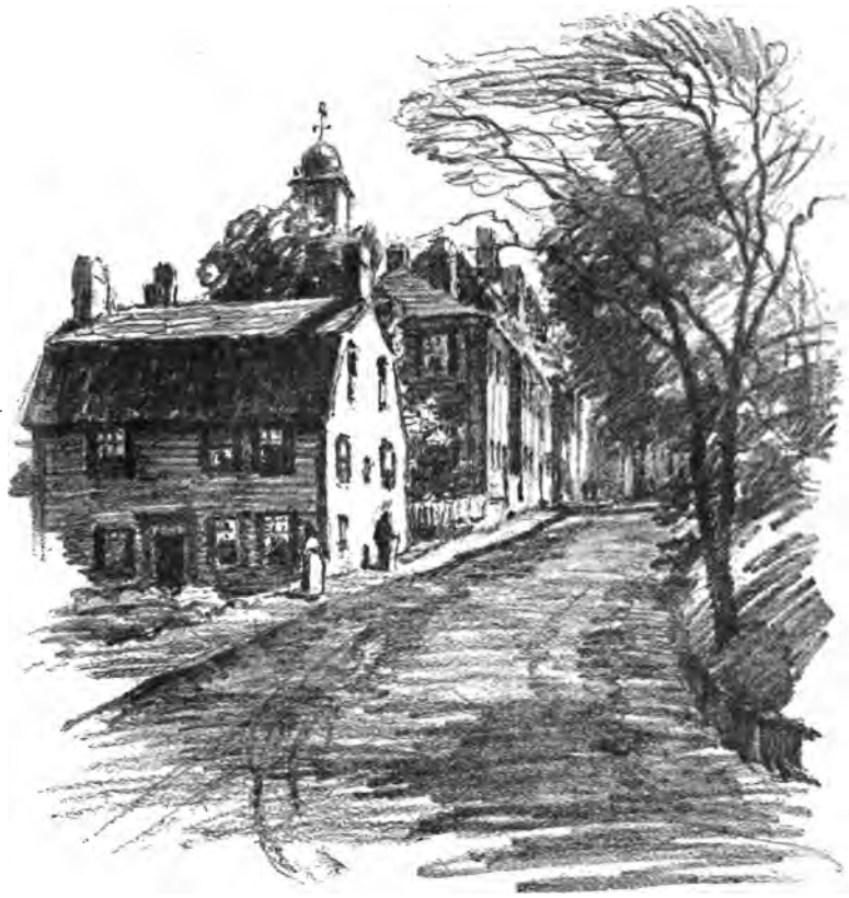
Site of First House, Leyden Street
